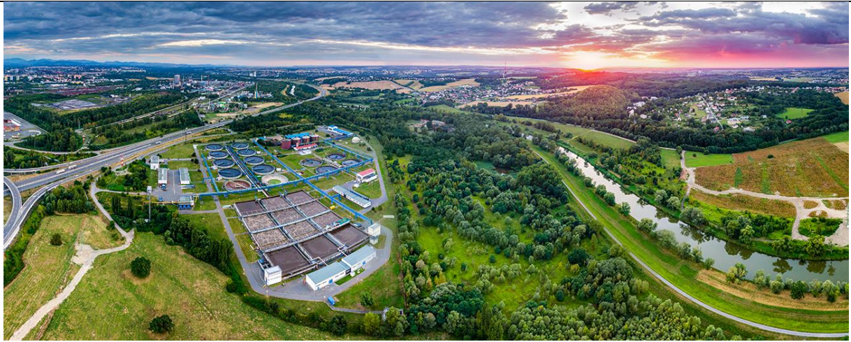
Image 2: Waste water treatment plant in Ostrava-Privoz
