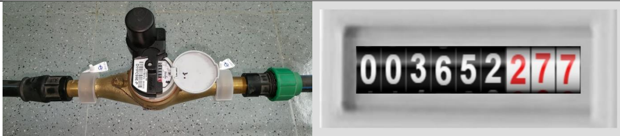
Image 5: Smart metering of water consumption
